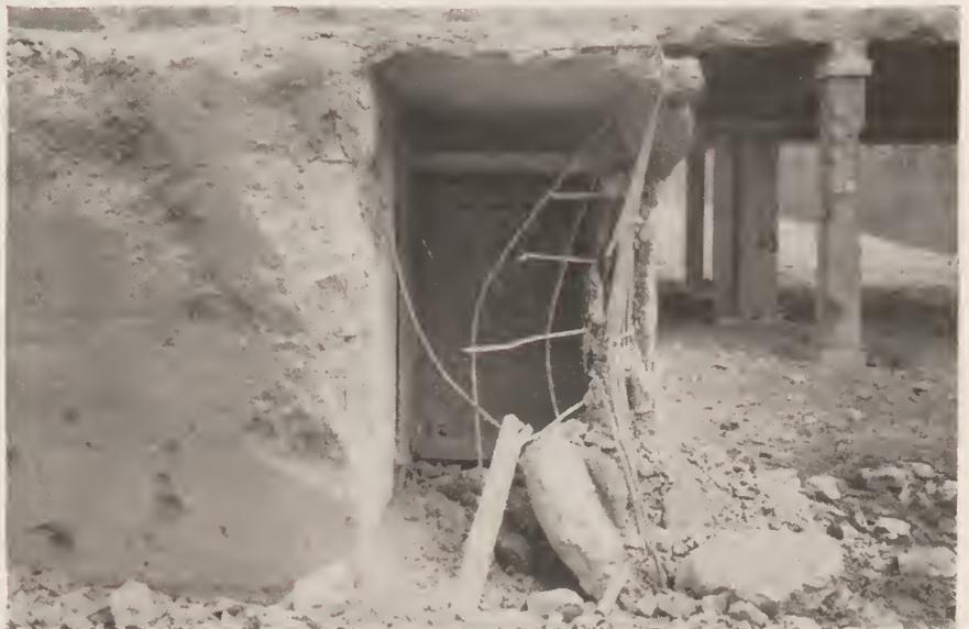
View of concrete surface shelter (No. 7) after completion of statically detonated bomb tests.
