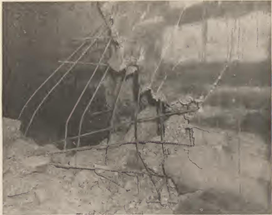
Bomb hit No. 46. Scabbing on north wall, lower story, section A of bombproof shelter B after hit in earth by 600-pound demolition bomb with delay-action fuse.
