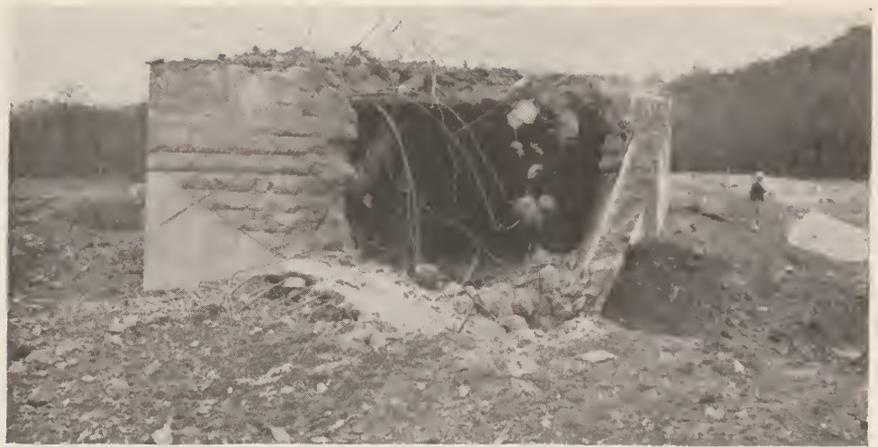
Bomb hit No. 47. Effects of hit on section C of bombproof shelter B made by 600-pound demolition bomb with delay-action fuse.
