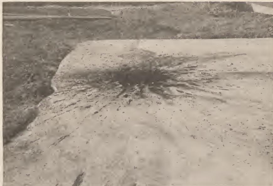
Bomb hit No. 16. Crater in burster slab No. 7 made by 100-pound demolition bomb with instantaneous fuse.
