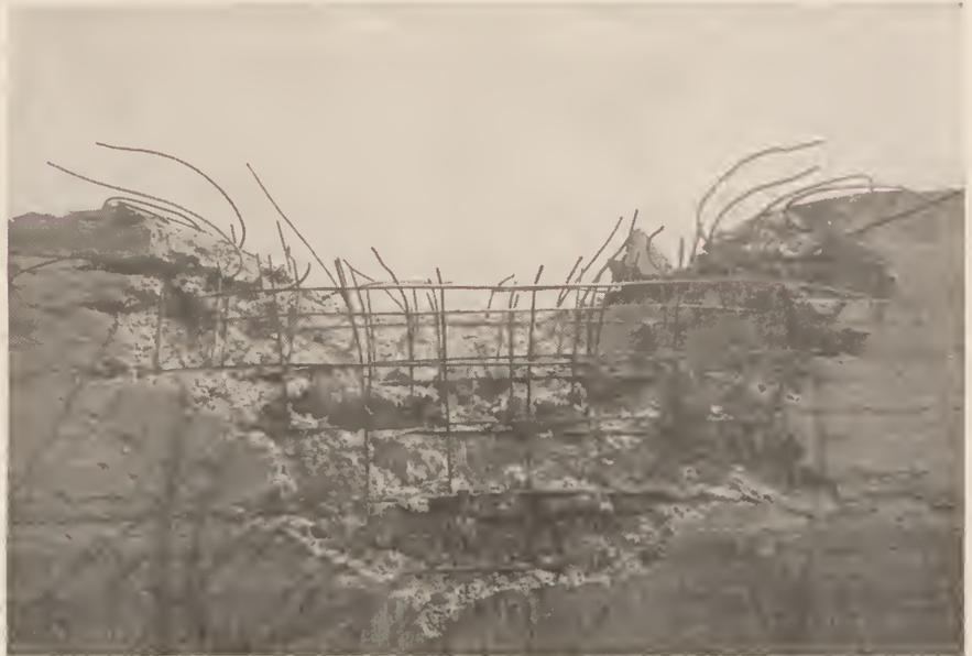
Bomb hit No. 44. Crater on roof, section A of bombproof shelter B made by 600-pound demolition bomb with delay-action fuse.
