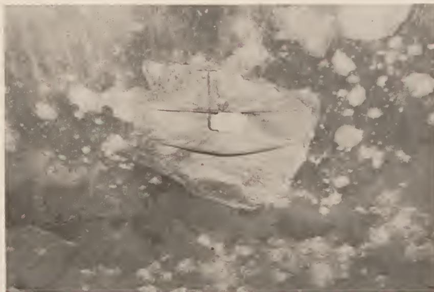
Bomb hit No. 15. View of scabbing underneath slab of section B of building prototype made by 100-pound demolition bomb with delay-action fuse.
