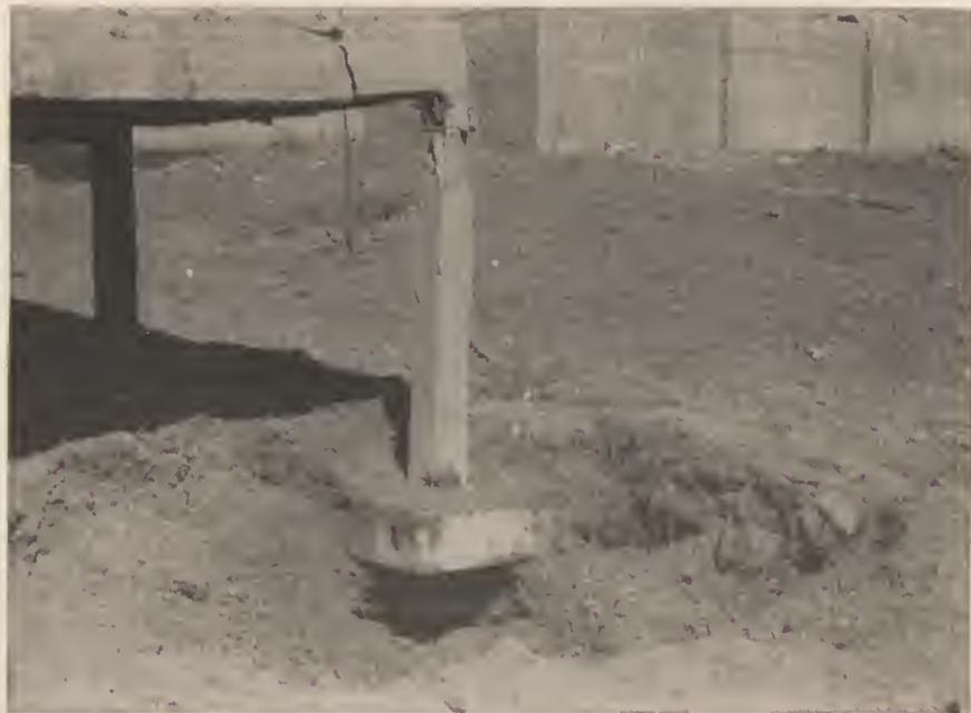
Bomb hit No. 5. Effects of hit in earth near section C of building prototype made by 100-pound demolition bomb with delay-action fuse.
