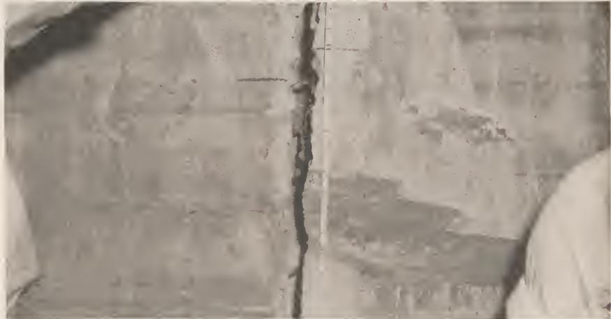
Bomb hit No. 43. Separation and vertical movement at construction joint. Sections B and C of bombproof shelter B after hit by 600-pound demolition bomb with delay-action fuse.
