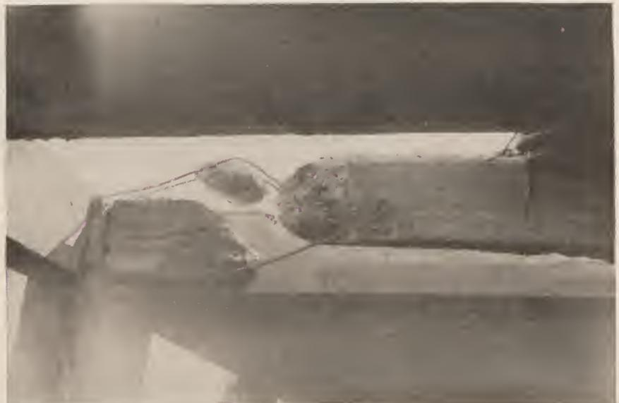
Bomb hit No. 3. Effects of hit on section A of building prototype made by 100-pound demolition bomb with delay-action fuse.
