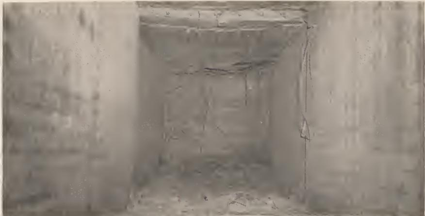
Bomb hit No. 47. Interior of south rooms, lower story of bombproof shelter B after hit by 600-pound demolition bomb with delay-action fuse.
