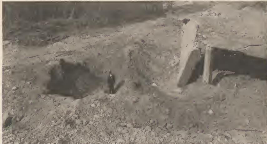
Bomb hit No. 38. Effects of hit in earth near section C of building prototype made by 600-pound demolition bomb with delay-action fuse.
