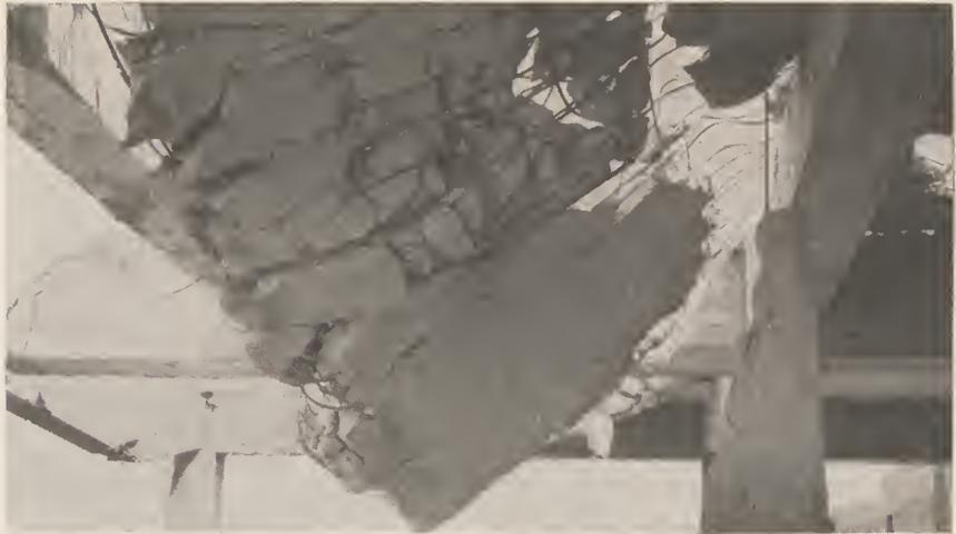
Bomb hit No. 9. Effects of hit on section A of building prototype made by 100-pound demolition bomb with delay-action fuse.
