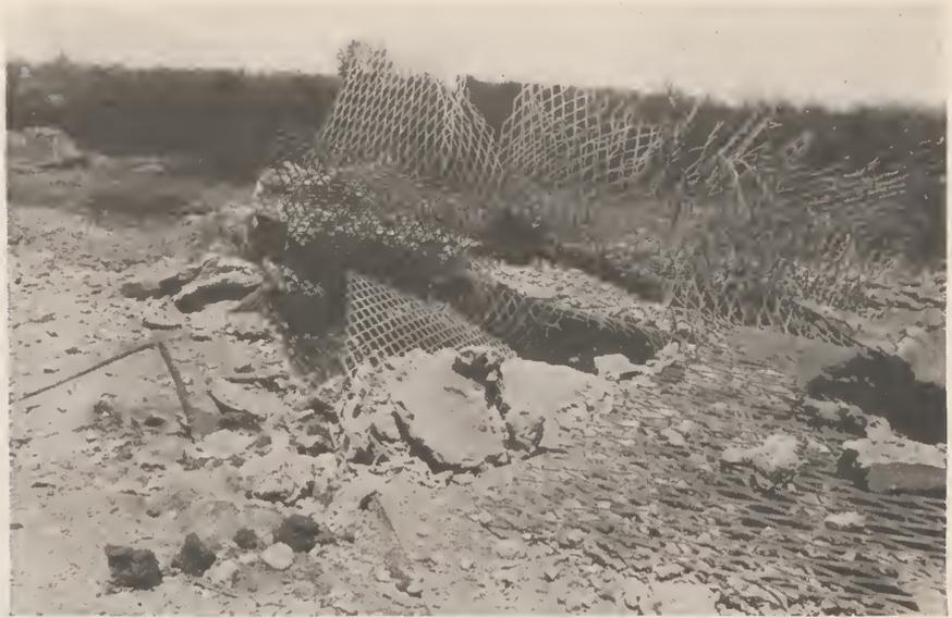
Bomb hit No. 32. Effects of hit on burster slab No. 3 made by 600-pound demolition bomb with delay-action fuse.
