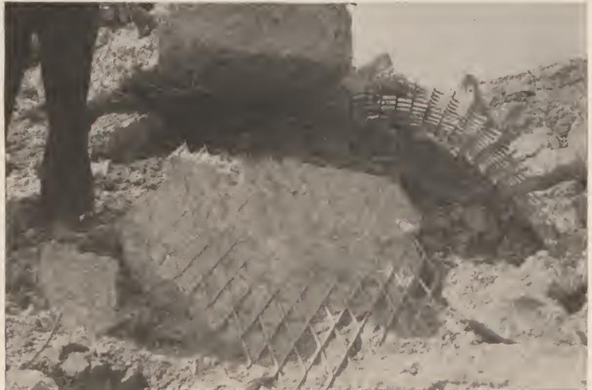
Bomb hit Nos. 36 and 37. Effects of hits on burster slab No. 3 made by 600-pound demolition bomb with delay-action fuses, illustrating laminar separation between concrete and expanded metal reinforcement.
