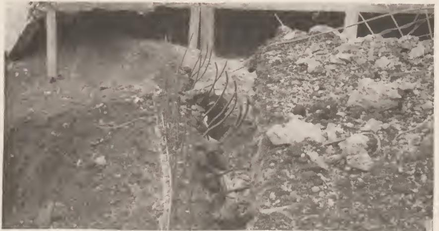
Bomb hit No. 47. Separation of roof and wall, section C of bombproof shelter B made by 600-pound demolition bomb with delay-action fuse.
