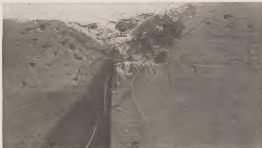
Bomb hit No. 31. Effects of hit on section A of bombproof shelter B made by 600-pound demolition bomb with delay-action fuse.
