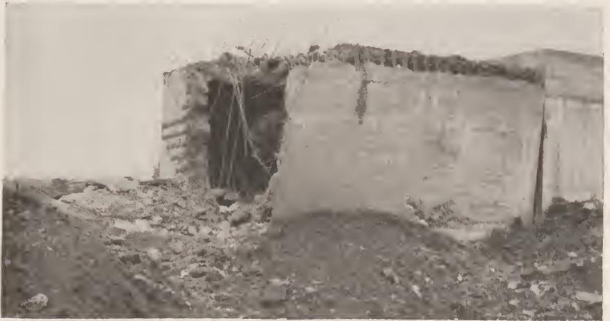
Bomb hit No. 47. Effects of hit on section C of bombproof shelter B made by 600-pound demolition bomb with delay-action fuse.
