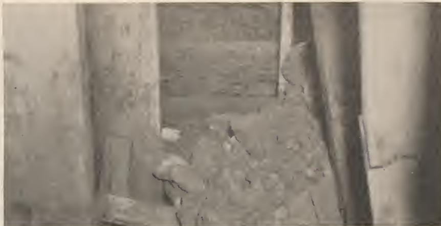
Interior of buried wood shelter (No. 2) after static detonation of 600-pound demolition bomb.
