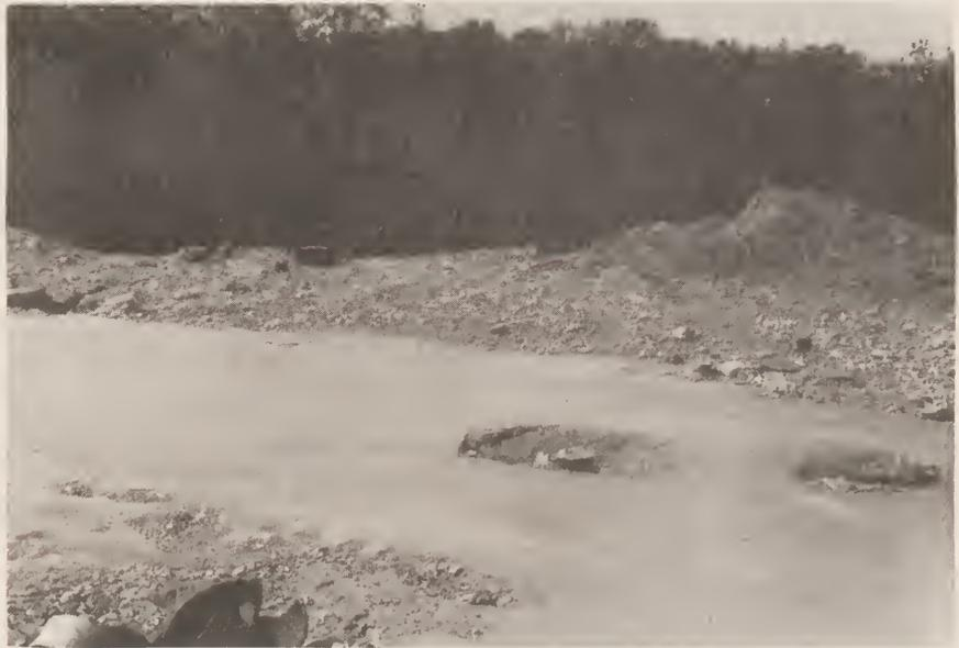
Bomb hit No. 30. Cracking in burster slab No. 2 made by 600-pound demolition bomb with delay-action fuse.
