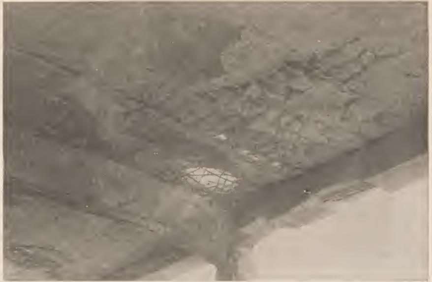
Bomb hit No. 24. Effects on reinforcing in section C of building prototype after hit by 300-pound demolition bomb with delay-action fuse on burster slab No. 6.
